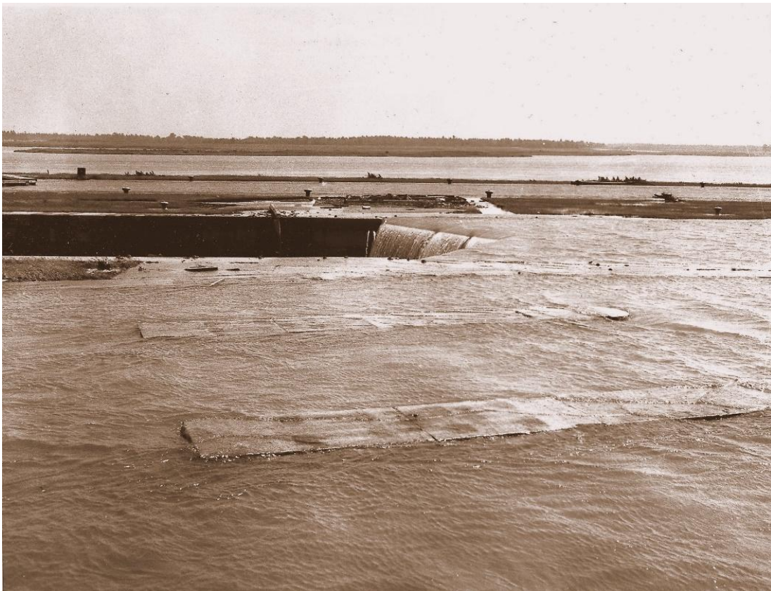
Flooding of Morrisburg Lock 23
